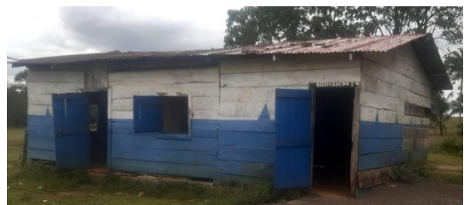
Existing classrooms (no longer in use)
